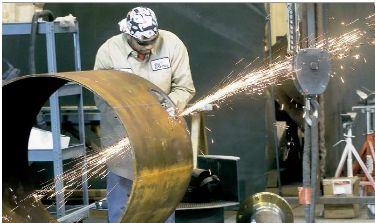
George Mayes, an Ely Energy code welder, adds a flange to a pressure vessel for a pollution abatement system Tuesday. SHERRY BROWN/Tulsa World
