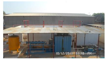
The SNG system shown is of 90 MMBTU/H @ 15 PSIG capacity designed by Aether dbs, USA. It has five Ventures which are shown below; two tanks in which mixture of water and glycol is filled and other parts of vaporizer are shown below.
