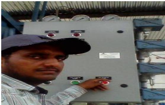
The shown picture is of the control panel that is used to turn ON the LPG transfer pump and as well as the indication came of any fault it can be reset by this panel.
