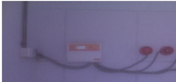
This is the control room of GT-System. There are four gas detectors which are placed in different places and their output hooters are connected.
