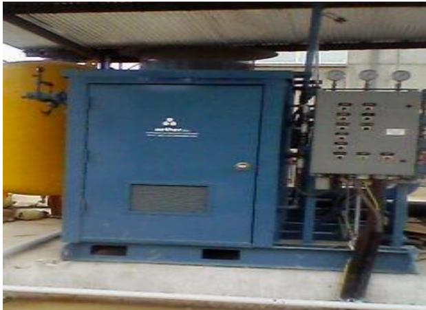
The SNG system shown is of 18 MMBTU capacity designed by Aether dbs, USA. It has one Venturi which is shown below; one tank in which mixture of water and glycol is filled and other parts of vaporizer is shown below.
