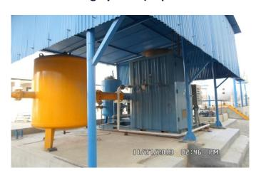
The SNG system shown is of 90 MMBTU/H @ 15 PSIG capacity designed by Aether dbs, USA. It has five Ventures which are shown below; two tanks in which mixture of water and glycol is filled and other parts of vaporizer are shown below.
